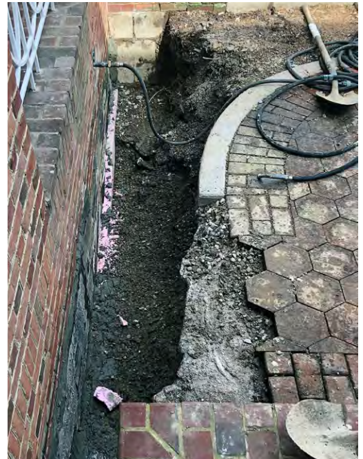
South breezeway deck pavers being re-laid and repointed for better waterproofing.
