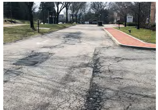
All of the asphalt parking lots and driveways on the property will soon be replaced.
